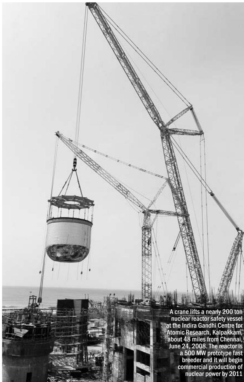
A crane lifts a nearly 200 ton nuclear reactor safety vessel at the Indira Gandhi Centre for Atomic Research, Kalpakkam, about 48 miles from Chennai, June 24, 2008. The reactor is a 500 MW prototype fast breeder and it will begin commercial production of nuclear power by 2011
